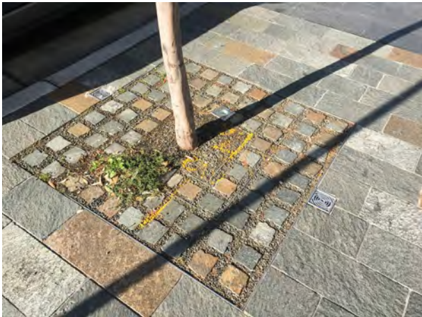
PORPHYRY STONE SETTS WITHIN AGGREGATE TREE PIT
